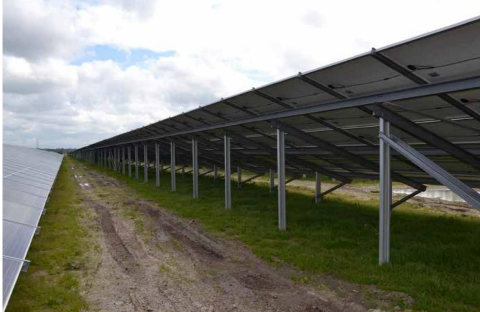
Image 2-1: Illustrative solar PV module (monofacial) on a mounting structure.
